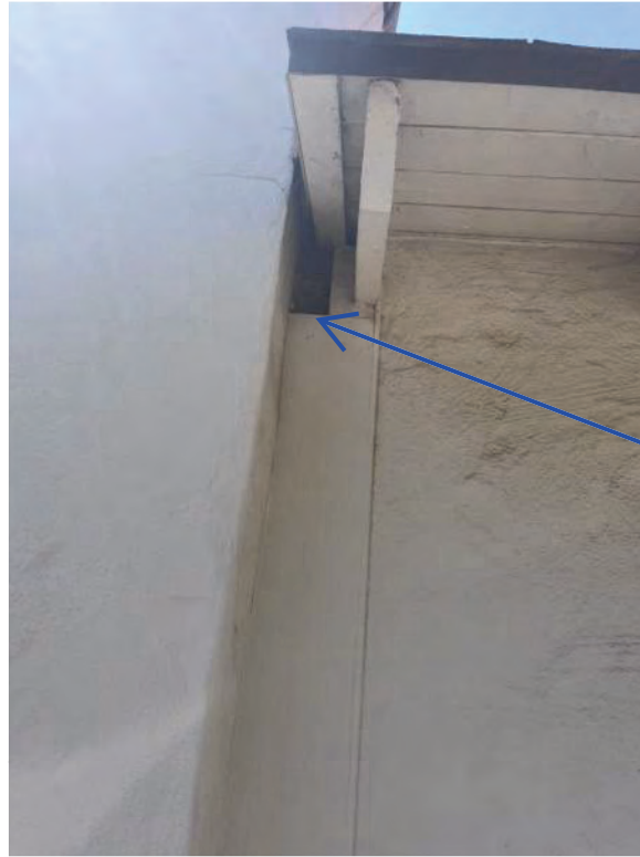
Clearance to Adjacent Structure
