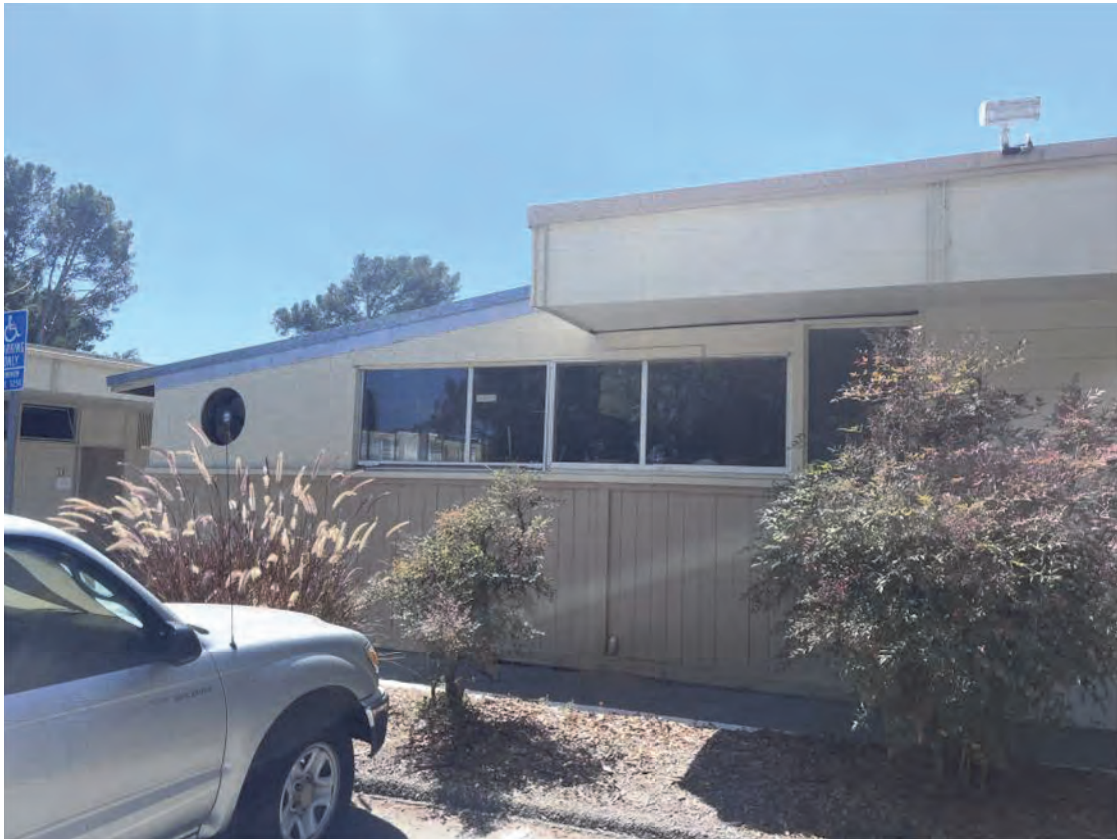
Addition @ South-East Corner - Exterior
