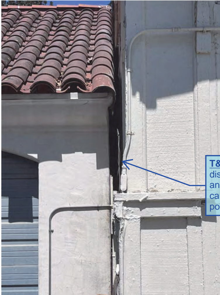
Clearance to Adjacent Structure
