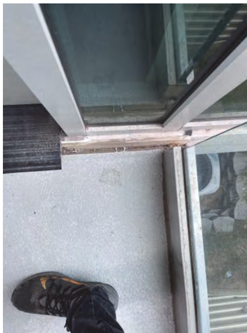
Seismic Separation @ Stair
