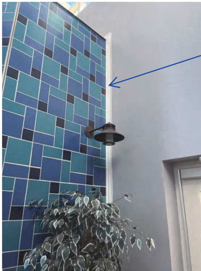
Seismic Separation @ 0007
