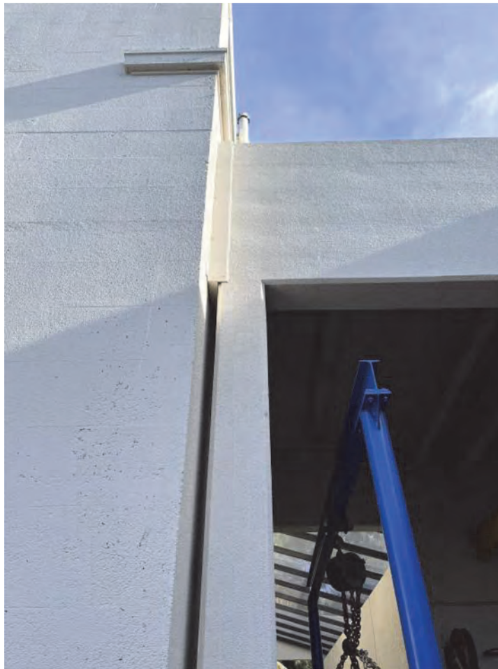
Seismic Separation @ 0001.1
