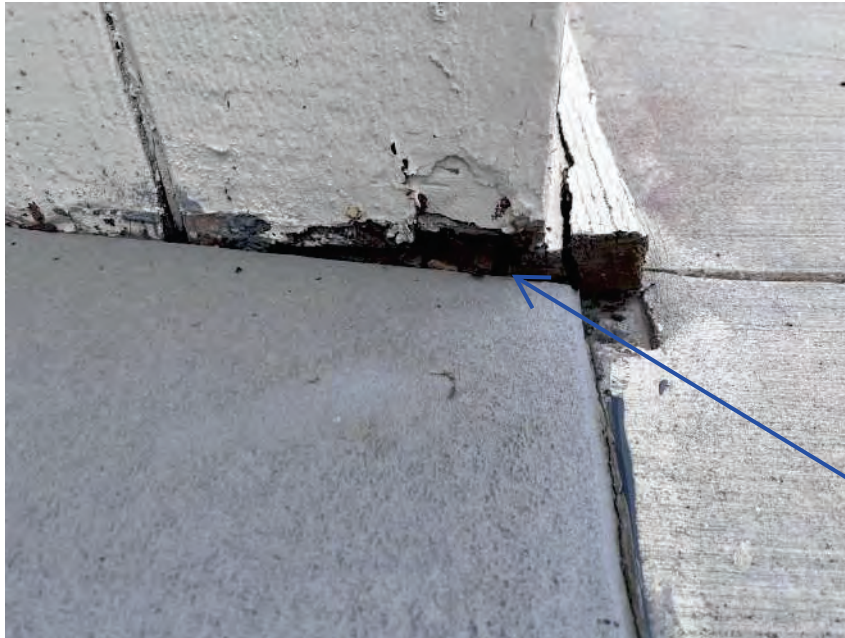
Pressure Treated Wood Sill-On-Ground
