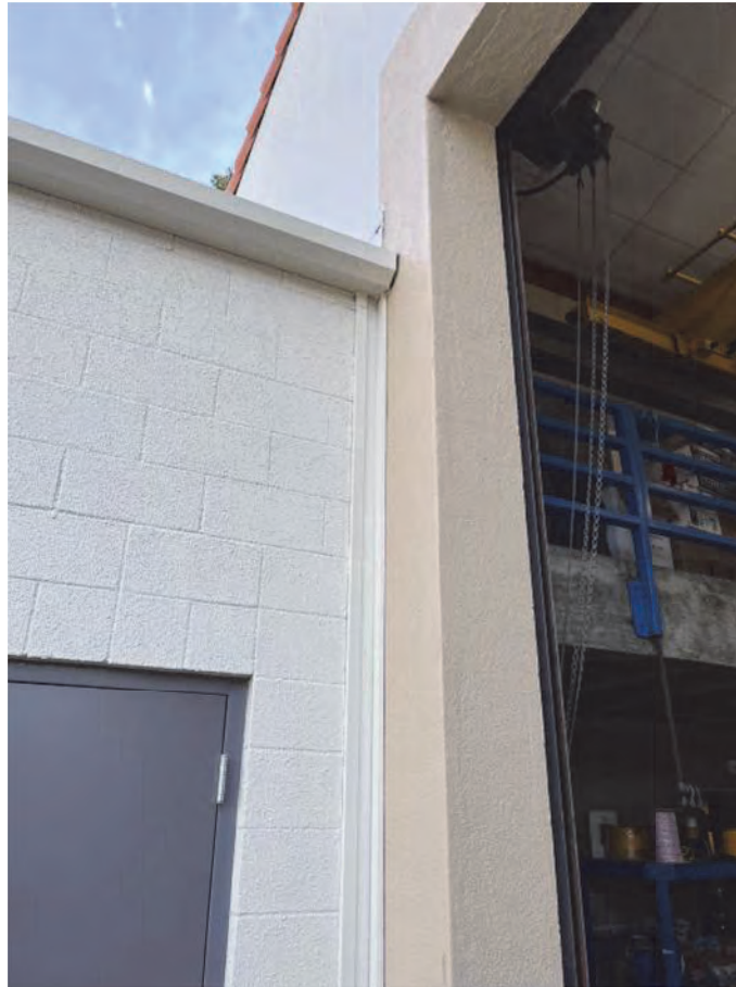
Seismic Separation @ 0016
