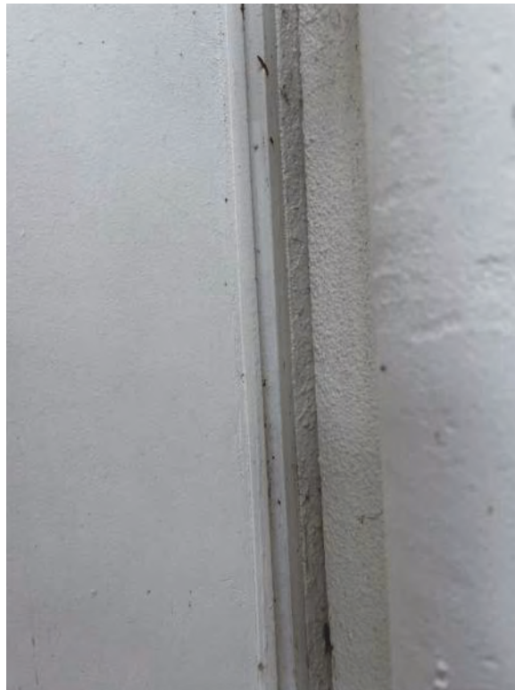
Seismic Separation @ Storage
