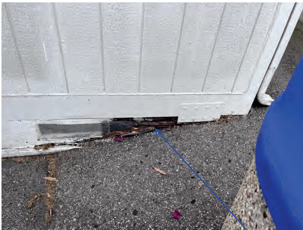
Pressure Treated Wood Sill and Rim
