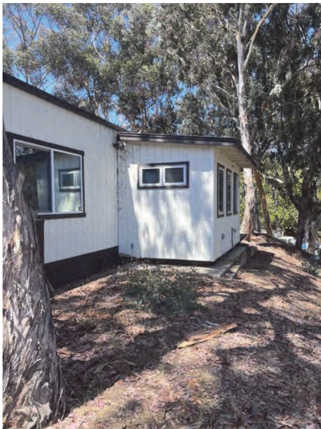
Single Room Addition to East Side
