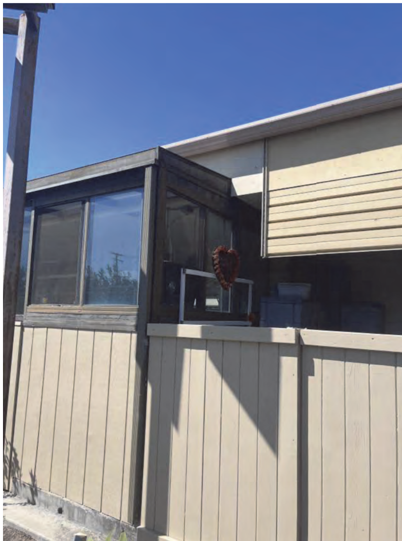
Addition @ South-West Corner - Exterior
