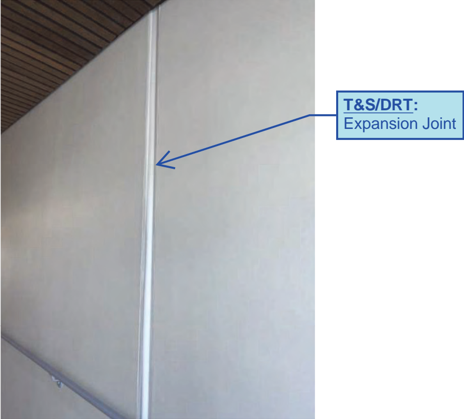
Seismic Separation @ 0007
