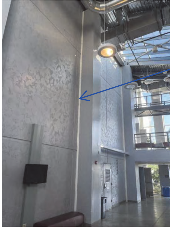
Seismic Separation @ 0007
