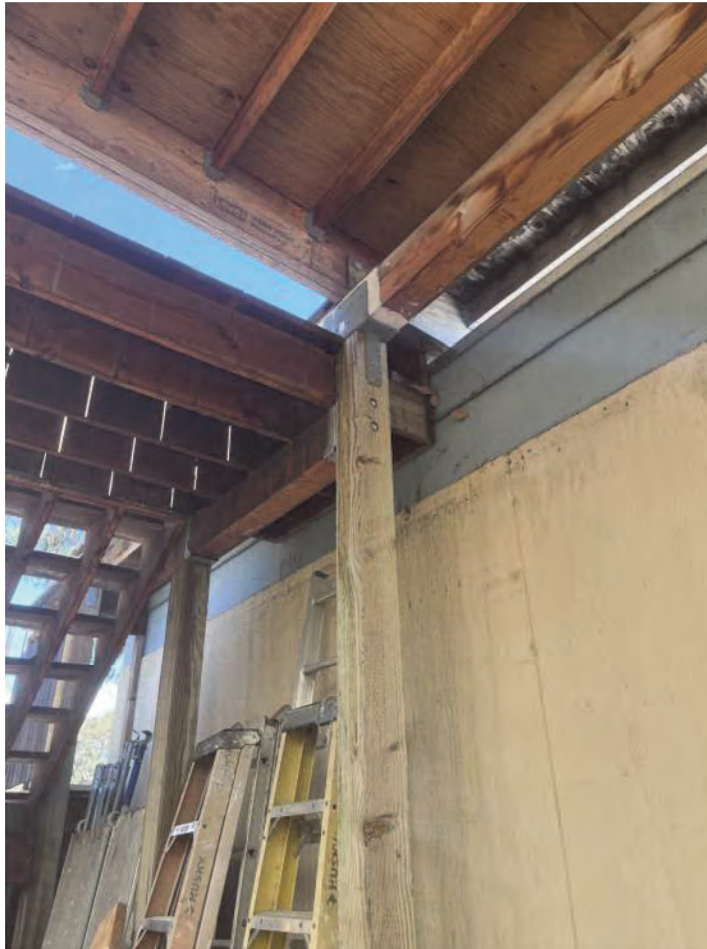
Stair, Landing, & High Roof Addition @ West Courtyard
