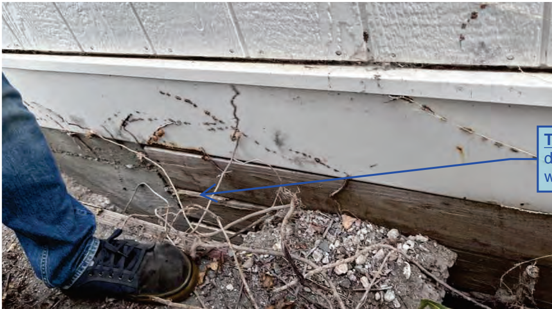
Wood Blockout for Sewage Drainage
