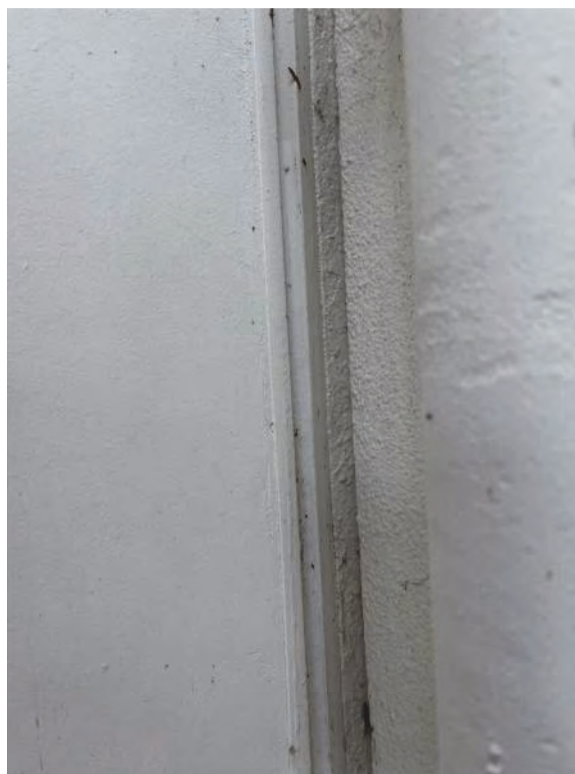
Seismic Separation @ Storage
