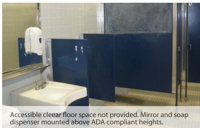
Compliant maneuvering clearances are not provided
