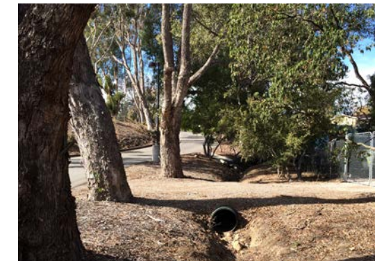
drainage ditch along northern edge of campus
