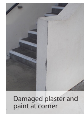
Exterior walls, peeling plaster paint
