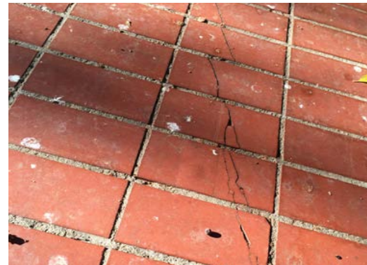
mortar set brick on concrete slab
