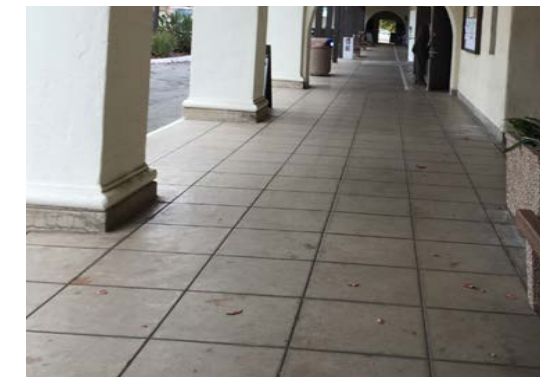
concrete arcade walk
